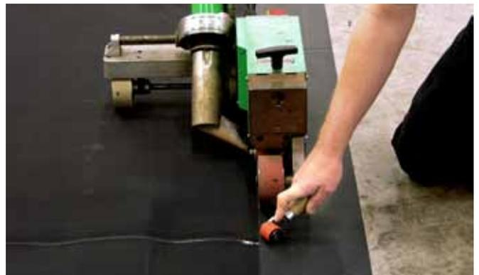
If the Thermobond strip is applied transverse to the membrane lengthway this creates a T-joint. The difference in level must be evened out with Hot melt sealant before bringing on the Thermobond strip as previous described. This areas shall be pressed with pressure roll after the splicing machine passes and re-heats the Hot melt sealant.
