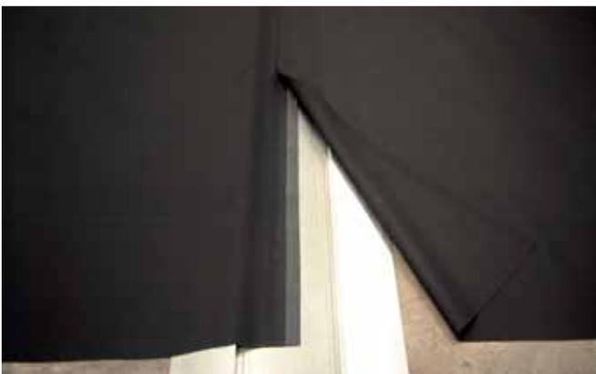
Position the second lengthway so that the overlap is aligned with the markings on the membranes that equal 70 mm overlap.
