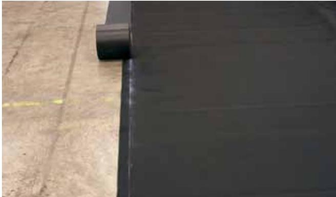
Mark out a 50 mm overlap on the panel and position the Thermobond strip.
