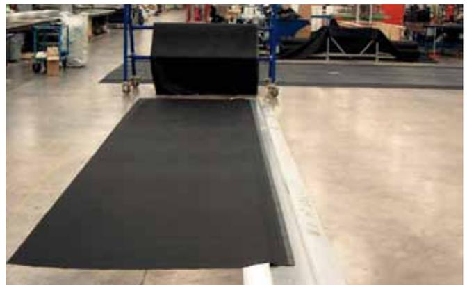
Unroll the first lengthway in required length with the grey Thermobond edge facing upwards, centred in the guiding trench.
