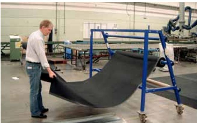
The positioning of the membrane is easier if the membrane is put in unrolling equipment that can be moved around.
