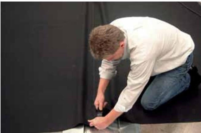
The hot wedge doesn't close the splice where it has started. Therefore the splice at the starting point shall be torn open until full strength is noted.
