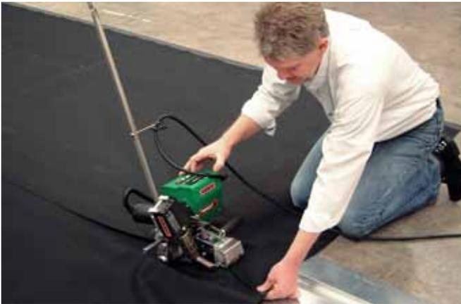
Place the Leister Twiny in position and insert the membrane. Stretch and hold the two layer of membrane when the machine starts.
