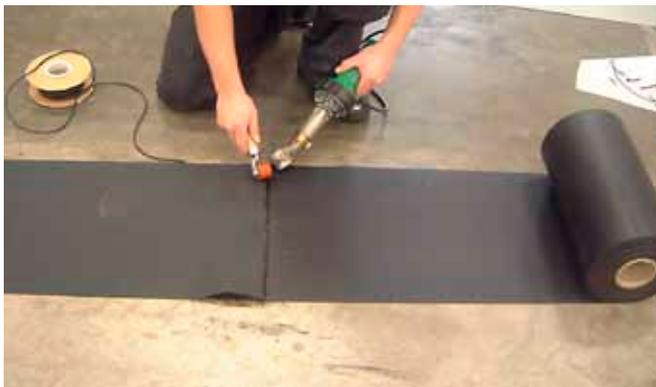
If the Thermobond splice strip must be prolonged this is done by overlapping the strips minimum 40 mm with the TPE facing upwards and splicing them together with Leister Triac. The difference in height must be levelled with Hot melt sealant where the strip should be spliced to a panel. The width of the hot melt sealant should be min. 50 mm.
