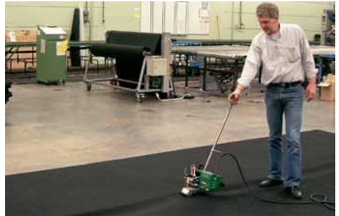
Always control and steer the machine as the splicing goes on. Sometimes the machine needs to be slowed down manually to avoid separation between the membranes.
