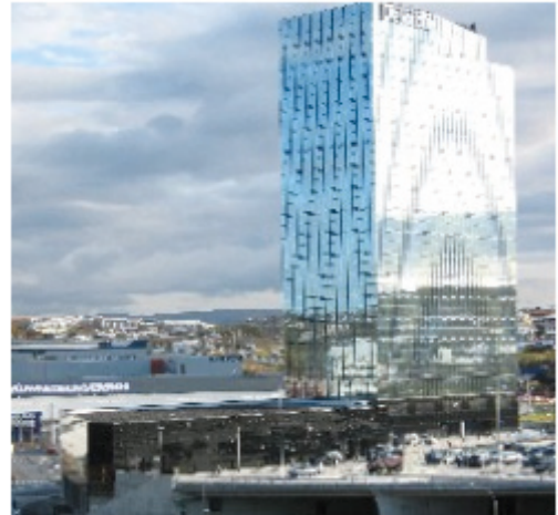
Smáratorg Tower, Reykjavik
